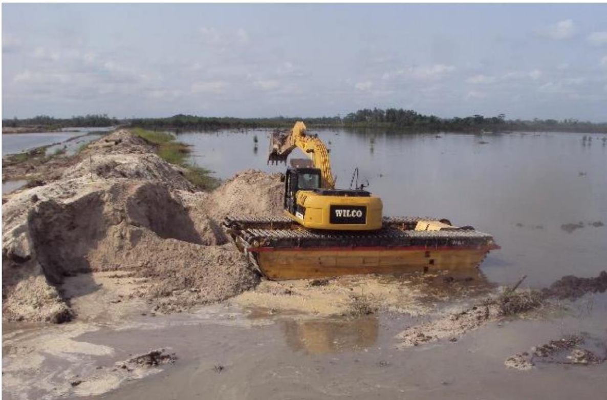
EXCAVATION AT SOKU WELL 56T 6" SECTIONAL REPLACEMENT. CLIENT SPDC
