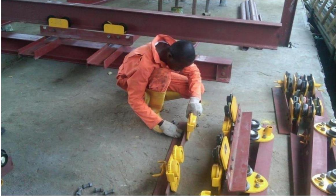
FABRICATED TROLLEYS FOR SANTA-BARBARA MPF LIFTING EQUIPMENT JOB. CLIENT: SPDC
