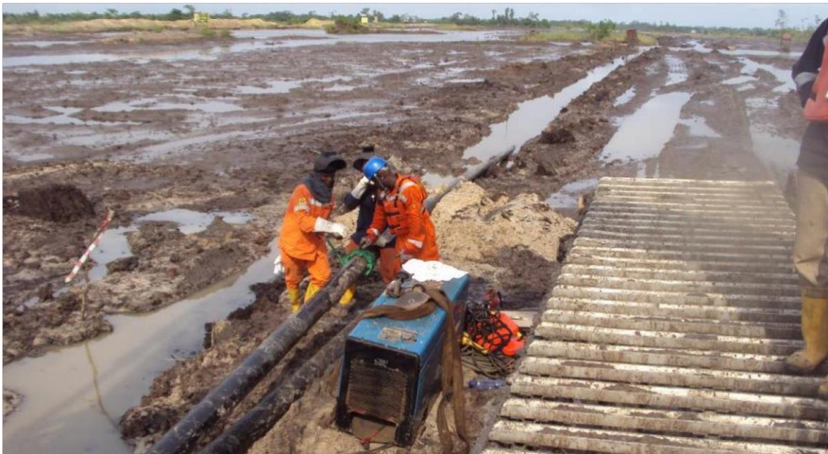
FLOW LINE TRACING AT SOKU WELL 56T 6" SECTIONAL REPLACEMENT. CLIENT SPDC TIE-IN AT SOKU WELL 56T 6" SECTIONAL REPLACEMENT. CLIENT SPDC
