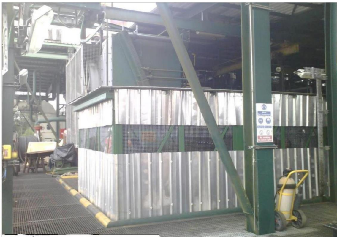
COMPLETED CHEMICAL SHED AT BELEMA AGG (INSIDE VIEW)
