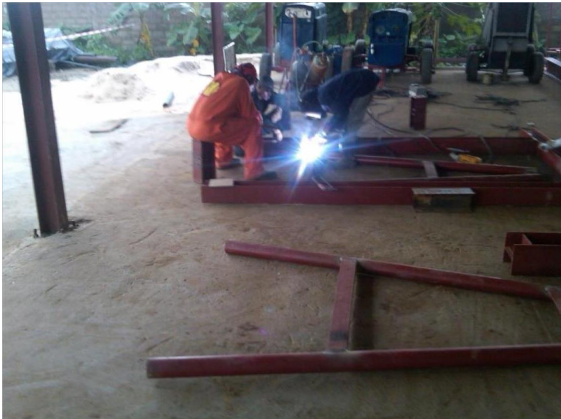
FABRICATION OF MOBILE GANTRIES IN PROGRESS FOR SANTA-B MPF LIFTING EQUIPMENT JOB. CLIENT: SPDC
