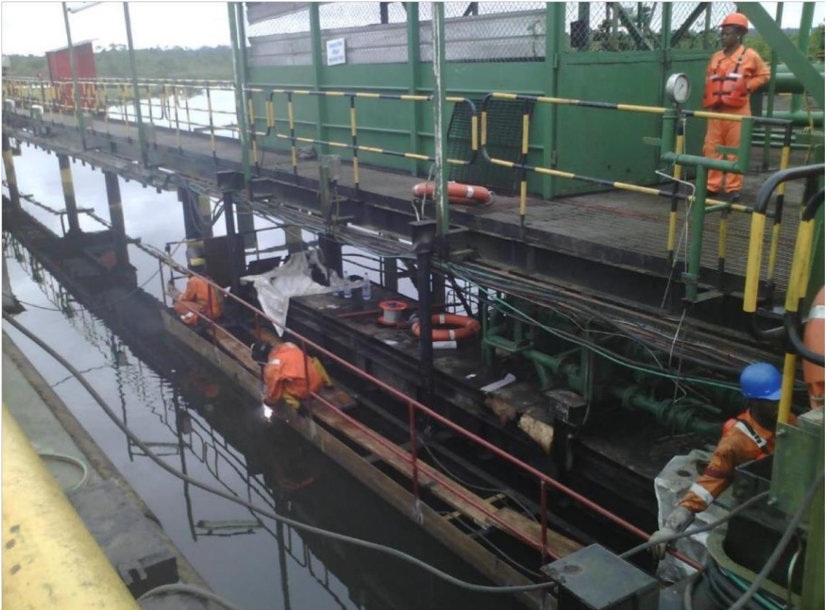
WELDING WORK AT SOKU W16L 4" SECTIONAL REPLACEMENT. CLIENT SPDC CONSTRUCTION OF BELEMA SAVER PIT FLOW STATION (CLIENT SPDC)
